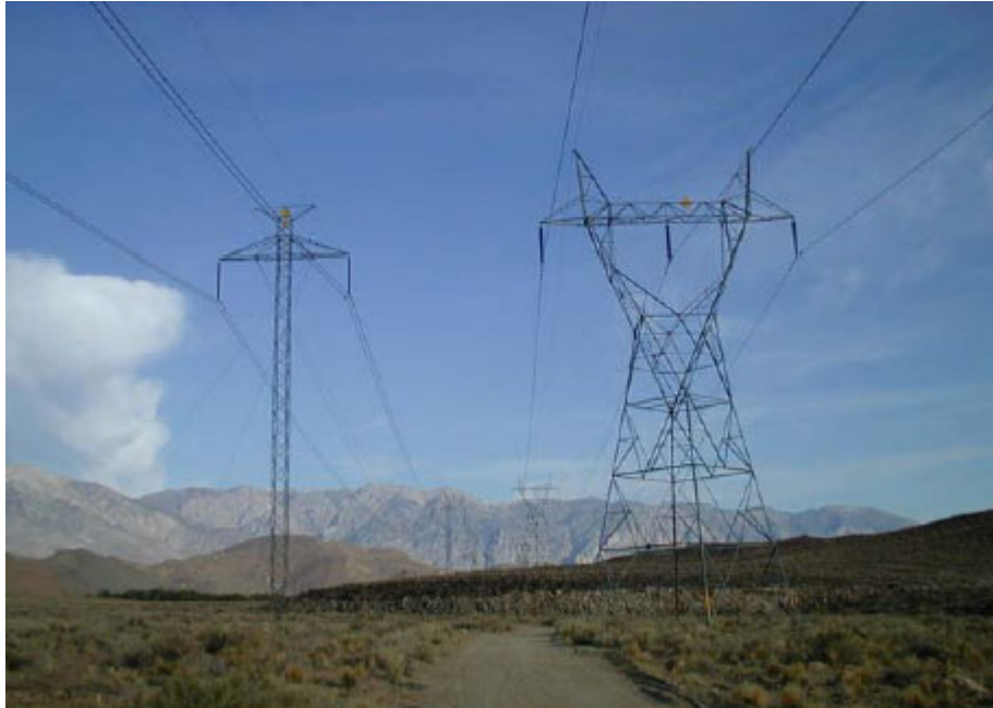
Figure 3. Comparison Left, power line: HVDC, 3,000 MW, +/- 500 kv bipole. Right, High Voltage AC 400 MW line. (Pacific Direct Current Intertie PDCI near Bishop, CA).
